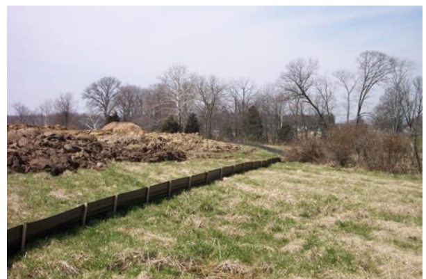
Figure 8 - Silt Fence (US EPA 2008)
