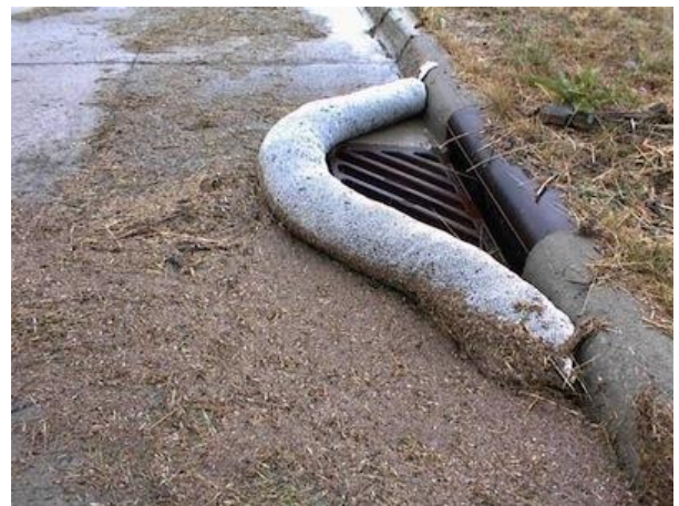
Figure 6 - Sediment Trap
