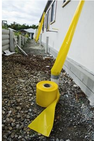
Figure 3 - Temporary Downpipes
