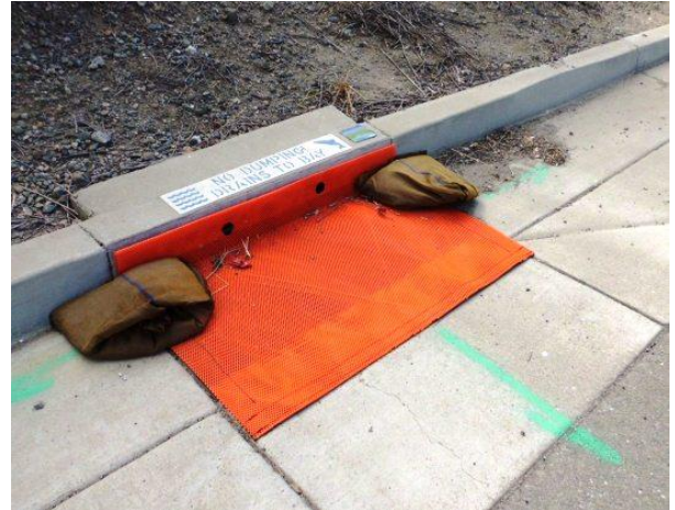
Figure 4 - Sediment Trap
