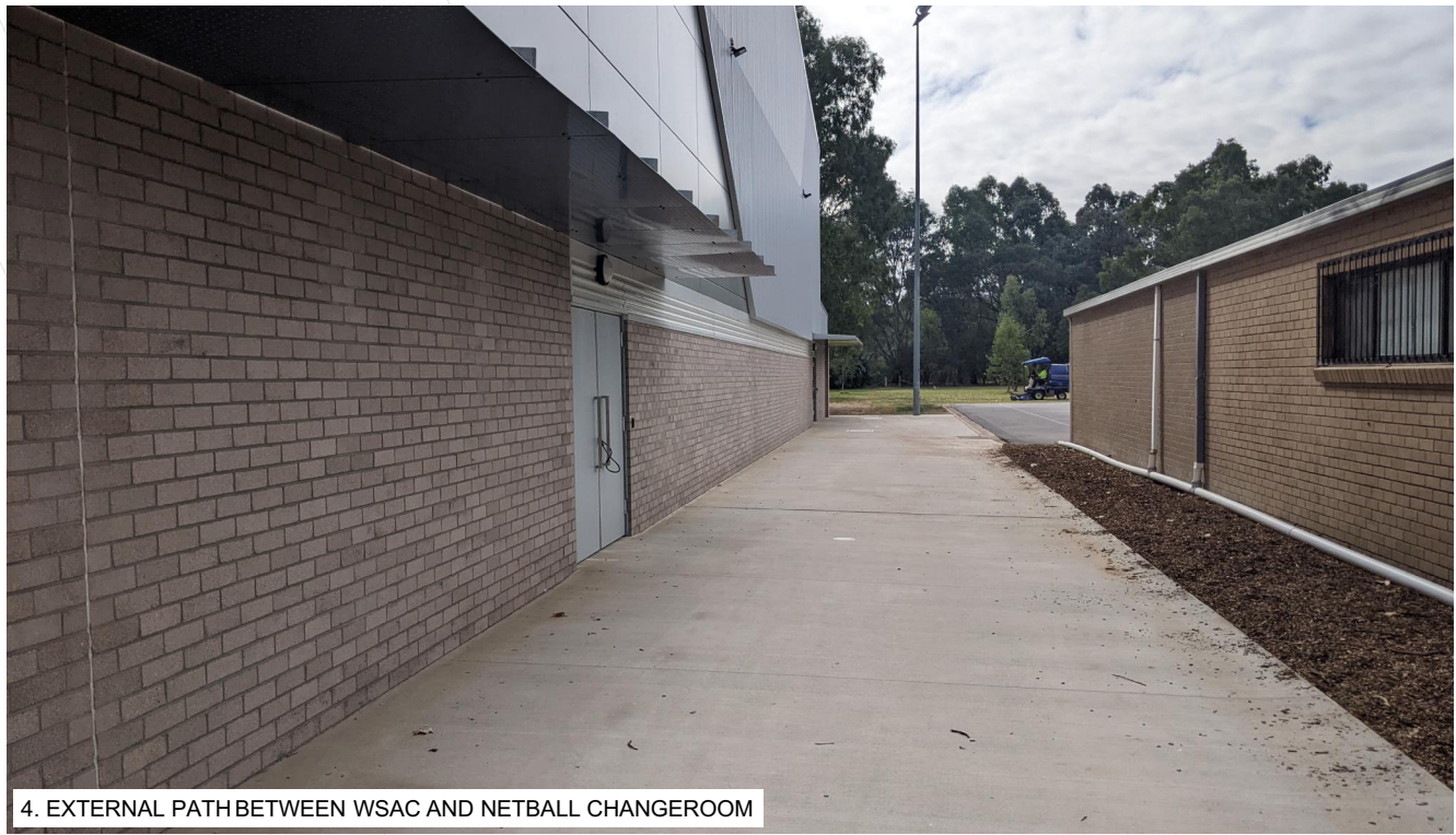
4. EXTERNAL PATH BETWEEN WSAC AND NETBALL CHANGEROOM
