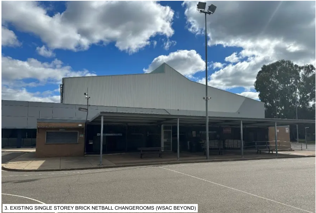
3. EXISTING SINGLE STOREY BRICK NETBALL CHANGEROOMS (WSAC BEYOND)
