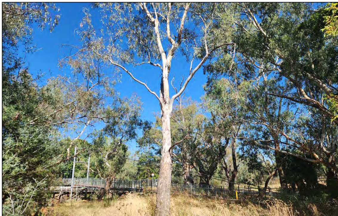
Photo 4: Zone 4. Looking west, towards pedestrian swing bridge. Photo: S. Mendham 2026
