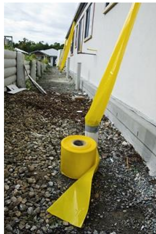
Figure 3 - Temporary Downpipes
