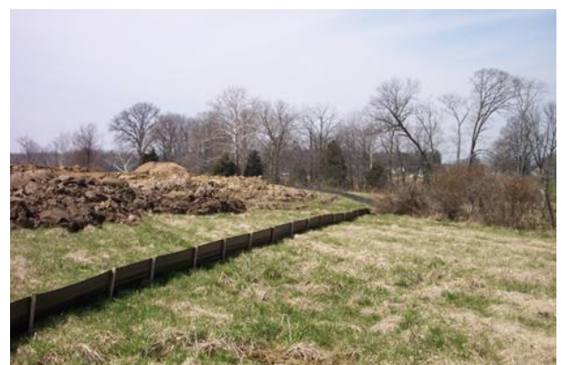
Figure 8 - Silt Fence (US EPA 2008)
